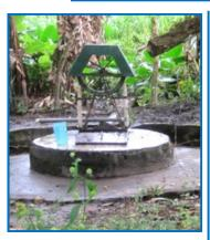
The above photo is the old San Diego well. which was constructed in 1992. The well has served as the primary source of water for the families that live in the area. However, the well is a shallow hand dug well, with a rope pump, and is located in a low lving area. The members of the committee indicated that the well is contaminated. most likely from infiltration of animal waste and other surface activities.
