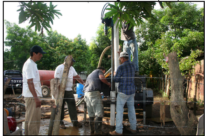
Putting in the casing, drilling is messy work!
