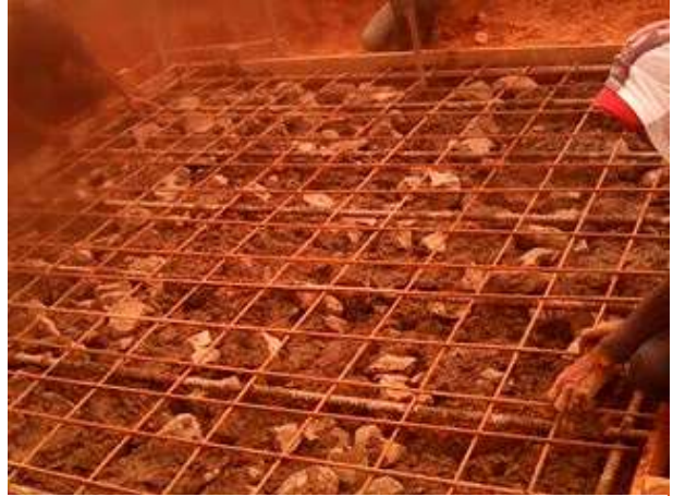
Construction of the base for the water tank
