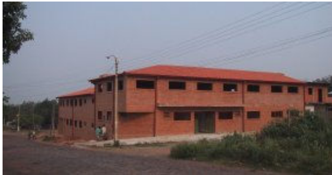
New Horizons School – Front View
