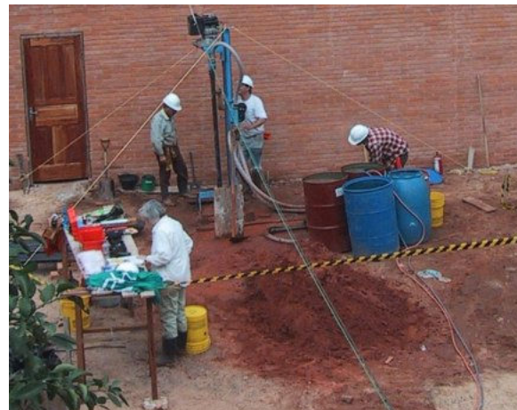
Drilling site view from above
