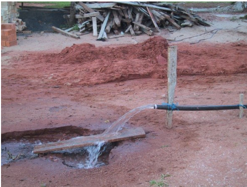
Water flowing after well was completed
