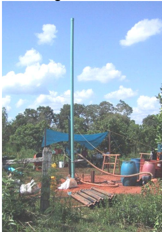
Installing PVC pipe in well
