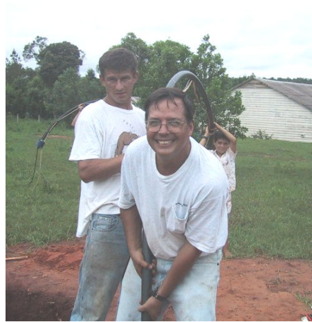
Ed & Dilio, plus children behind, installing pipe for pump
