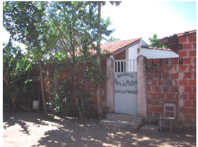
Entrance into the kindergarten
