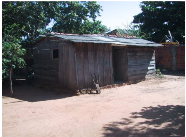
Parsonage at Santa Rosa Methodist Church
