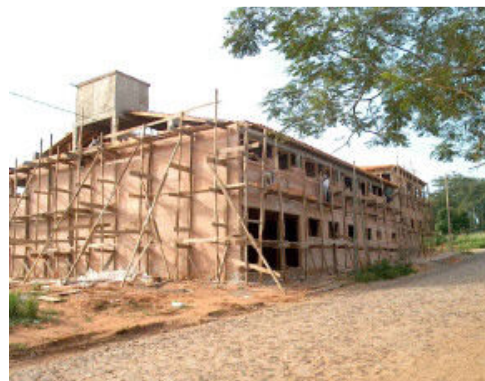
Methodist school under construction
